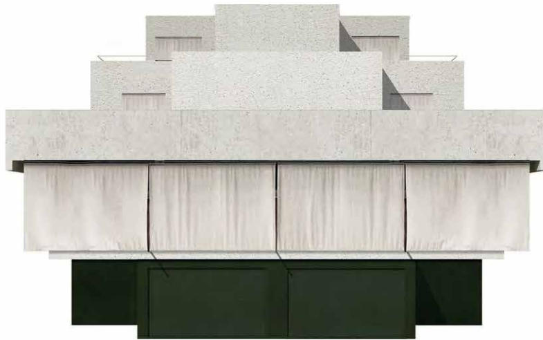
Residential building - Oberwil
